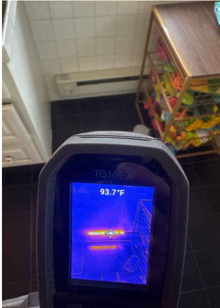
2nd Floor Bathroom
