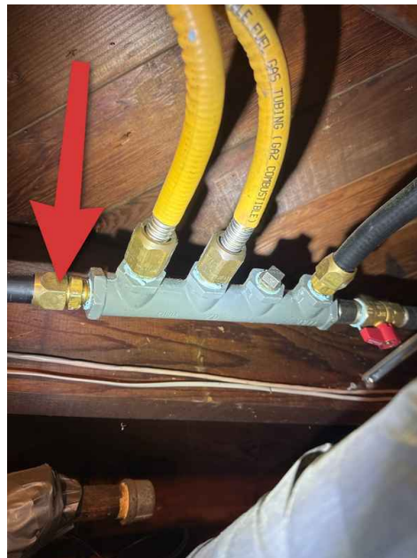
Illustration of proper bonding of CSST
