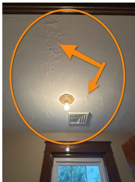
2nd Floor Front Office
