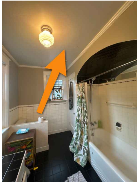
2nd Floor Bathroom
