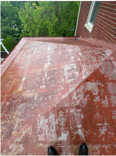
Right Side roof
