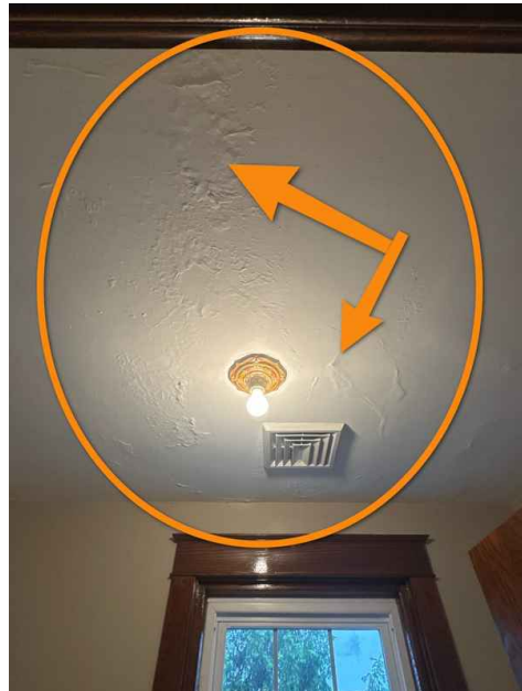
2nd Floor Front Office
