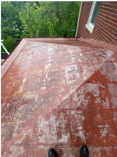
Right Side roof
