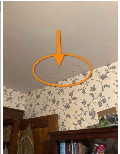
2nd Floor Front Right Side Bedroom
