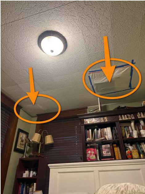
1st Floor Rear Right Side Bedroom
