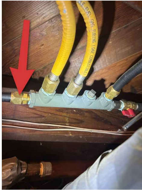
Illustration of proper bonding of CSST
