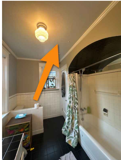
2nd Floor Bathroom
