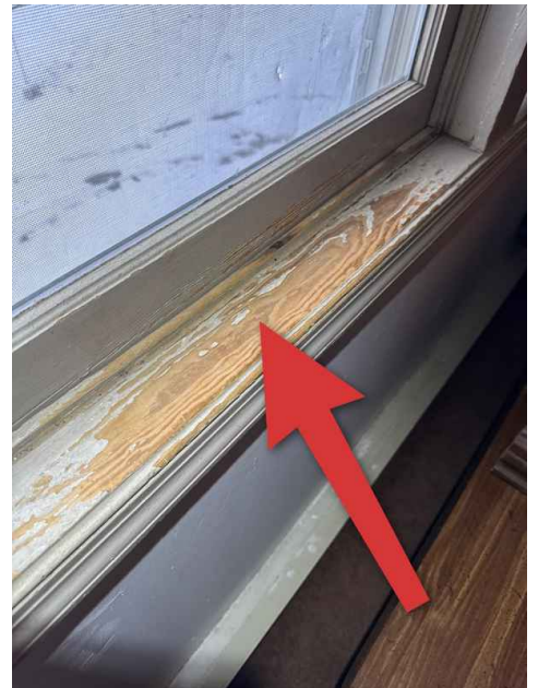
Significantly worn window sill
