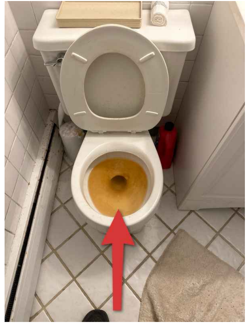
2nd Floor Hall Bathroom
