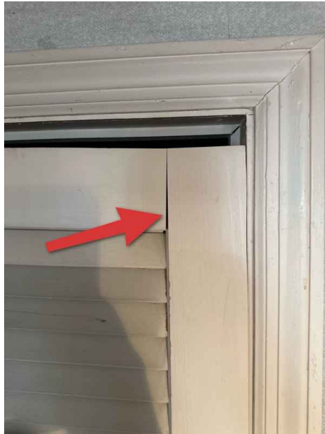
Close up split joint
