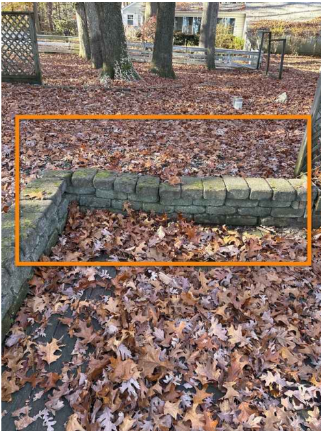
Rear retaining wall
