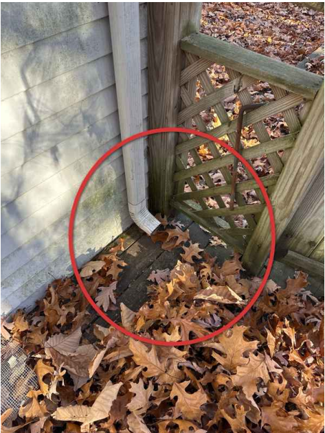
Rear Corner Garage
