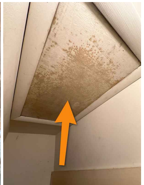
Attic access panel
