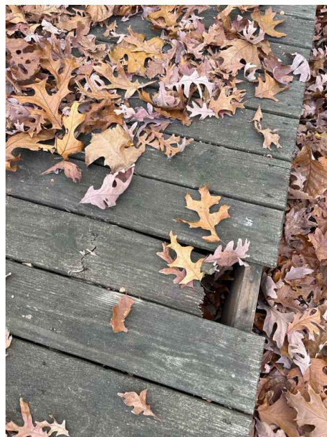
Damaged decking
