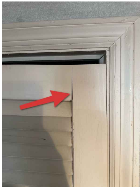
Close up spilt joint
