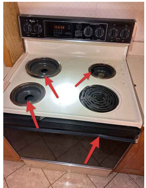
Missing elements and dented handle
