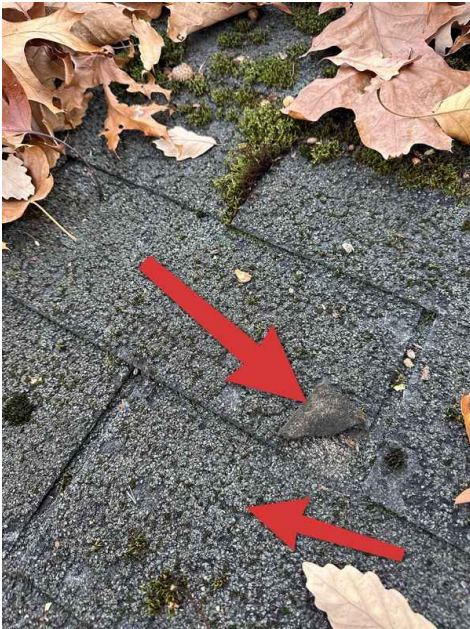
Brittle and cracked shingles
