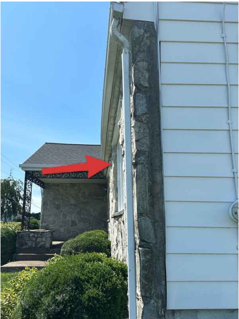
Front Wall Exterior
