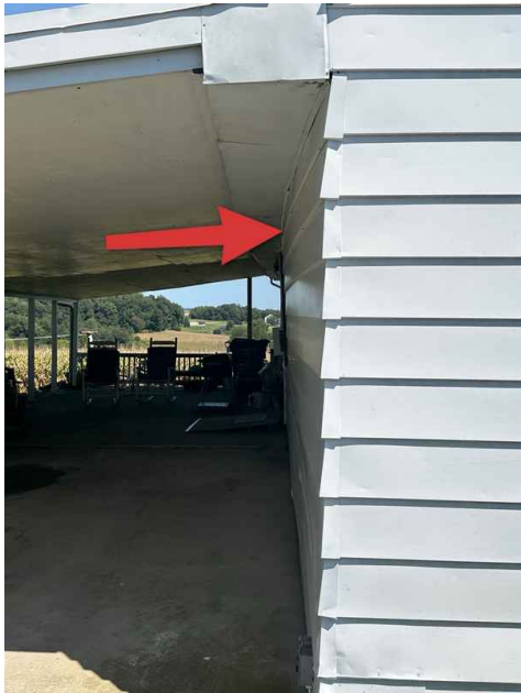
Rear Wall Exterior
