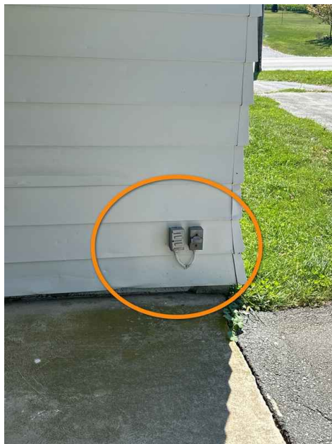
Rear Corner Carport
