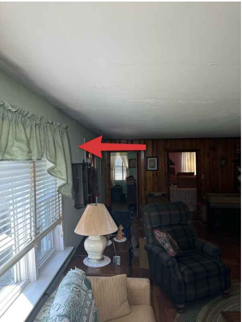
Front Wall Interior
