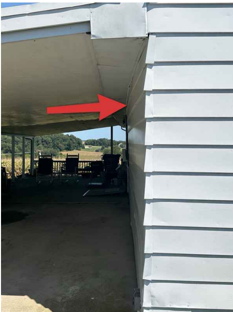
Rear Wall Exterior
