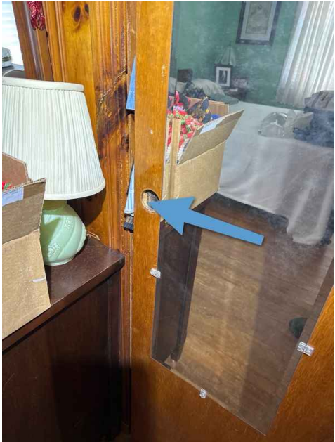
Front Bedroom Closet
