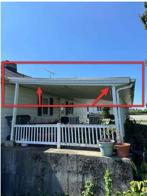
Porch ceiling and support structure
