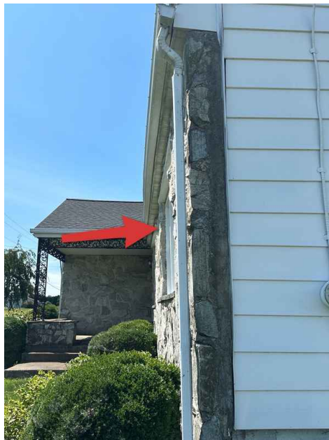
Front Wall Exterior
