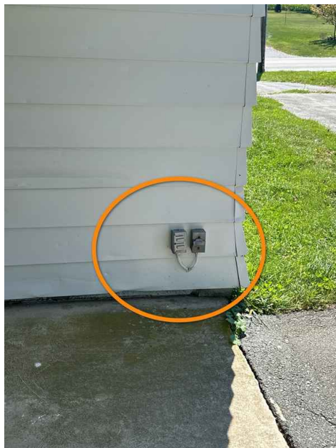
Rear Corner Carport
